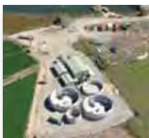
AquaMB Process® Multiple Barrier Membrane System
