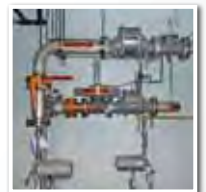
Pressure Regulator Flame Trap Assembly
