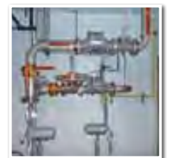
Pressure Regulator Flame Trap Assembly
