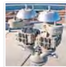
P/V Vent, Flame Arrester & Safety Selector Valve
