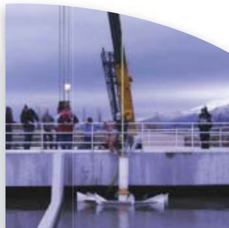
Rebuilds and BNR Upgrades
