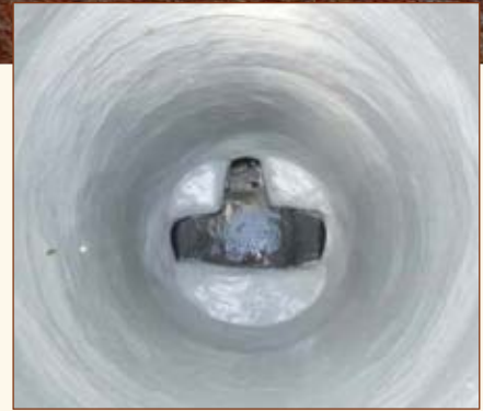
This sewer manhole was ravaged by H 2 S then structurally restored with Manhole Mortar™ and coated with 100% solids epoxy to prevent future corrosion and protect exposed concrete surfaces.
