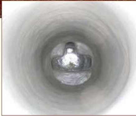
This sewer manhole was ravaged by H 2 S then structurally restored with Manhole Mortar™ and coated with 100% solids epoxy to prevent future corrosion and protect exposed concrete surfaces.
