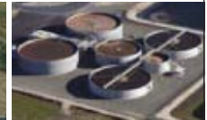
Anoxic & Nitrification Digester Tanks
