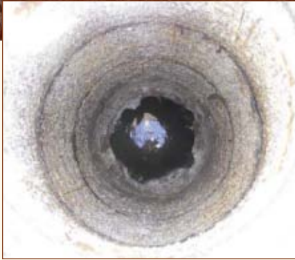
This sewer manhole was ravaged by H 2 S then structurally restored with Manhole Mortar™ and coated with 100% solids epoxy to prevent future corrosion and protect exposed concrete surfaces.
