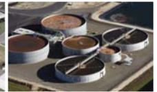
Anoxic & Nitrification Digester Tanks
