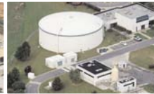
Storm Water Tank
