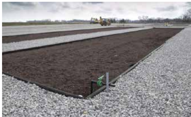
Figure 1 SAGR provides year round nitrification and effluent polishing
