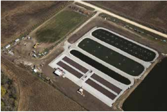
Figure 2 Aerial View of the Walker, IA WWTF in 2012.
