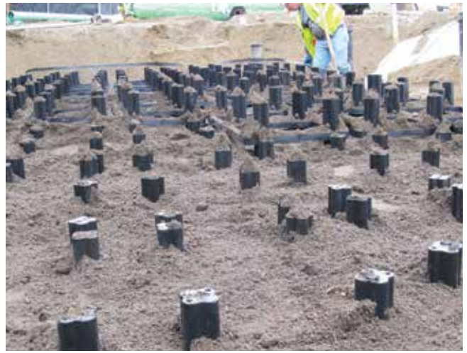
Left: Silva Cells are filled with soil for tree roots and on-site bioretention. Right: Silva Cells are filled with soil for tree roots and on-site bioretention. Photos courtesy of DeepRoot Green Infrastructure, LLC.
