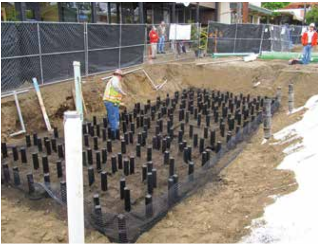
Left: Silva Cells are filled with soil for tree roots and on-site bioretention. Right: Silva Cells are filled with soil for tree roots and on-site bioretention. Photos courtesy of DeepRoot Green Infrastructure, LLC.
