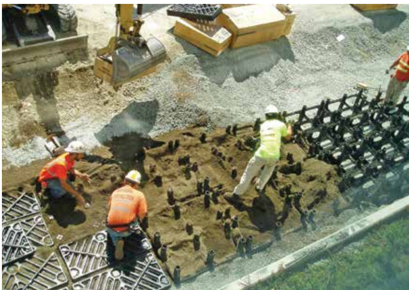
Aurora Avenue Project (Shoreline, WA)
