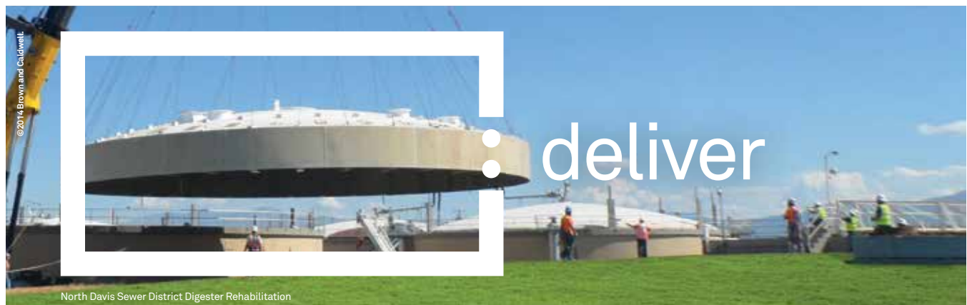
North Davis Sewer District Digester Rehabilitation
