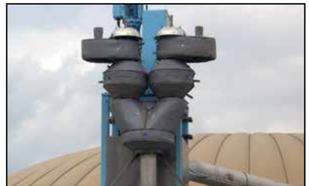
3-Way Safety Selector Valve with Combination Conservation Vents and Flame Arresters with Insulation Jackets
