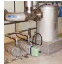
Sediment Trap with Electrically Actuated and Manual Drip Traps
