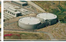
Equalization Tanks
