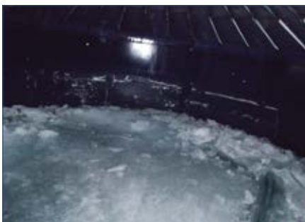
Frozen NY bolted tank
