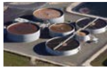
Anoxic & Nitrification Digester Tanks
