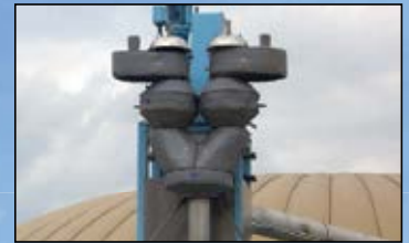
3-Way Safety Selector Valve with Combination Conservation Vents and Flame Arrester with Insulation Jackets
