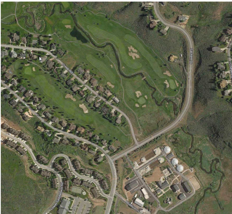
Aerial view of the Snyderville Basin Water Reclamation District that was captured from Google Earth.
