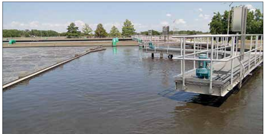
Using anoxic zones in the aeration basin improves energy efficiency at the Village Creek Water Reclamation Facility. (Credit: Kristina Twigg)
