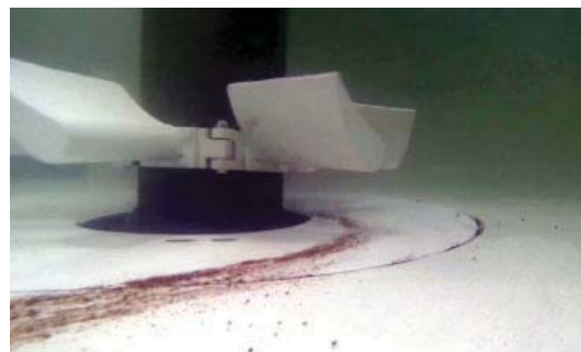
This underwater image demonstrates how incoming grit efficiently sweeps along the grit chamber's flat-floor for easy removal.
