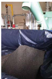
The grit system is removing 99 percent of the plant's incoming grit even during wet weather events.
