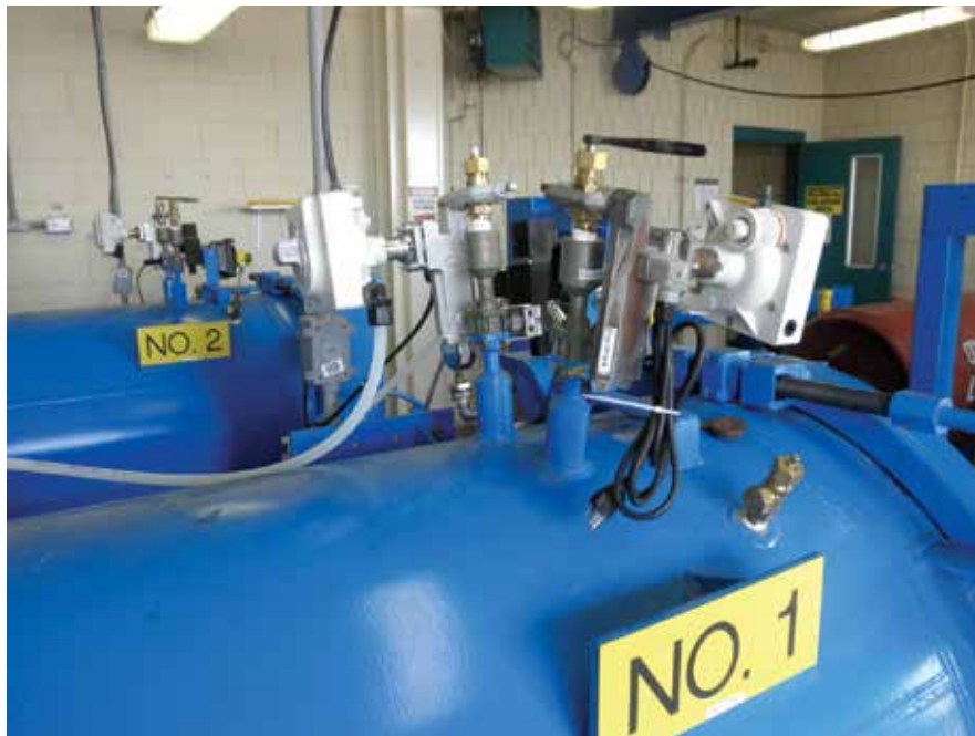
Innovative ChlorTainer™ cylinder containment vessels are designed for not less than 40 years of service. They enclose chlorine gas cylinders, the chlorine transfer hose, and seismic lock-down brackets. Vacuum breaker regulators are attached for fail-safe shutdown if there is a leak downstream.
