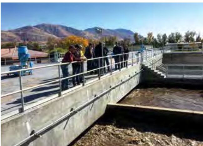
Figure 2. The group hears how the facility uses biological phosphorus removal to achieve < 0.5 mg/L total phosphorus.
