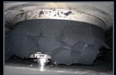
Dewatered Anaerobic Biosolids
