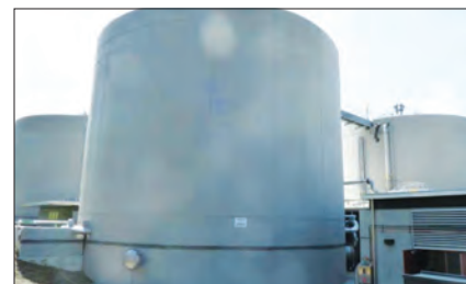
Figure 3: Modified “Silo” Type Digesters Mimic Egg-Shape Tanks
