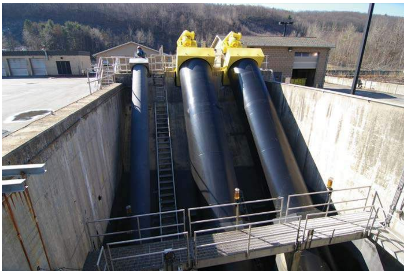
Lakeside's enclosed screw pump (left) and its twin screw pumps used for storm duty.
