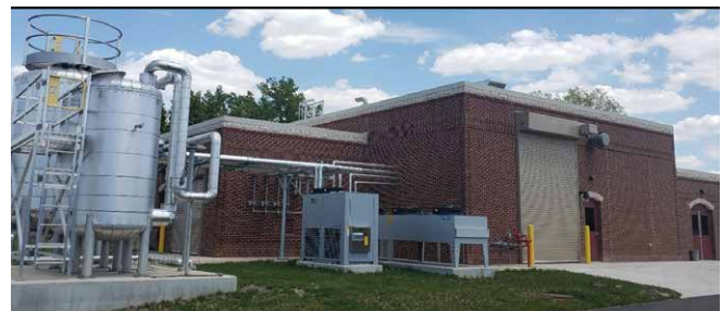
Until the Lakeside SAP was installed, the KWRD’s screens would regularly become blinded.
