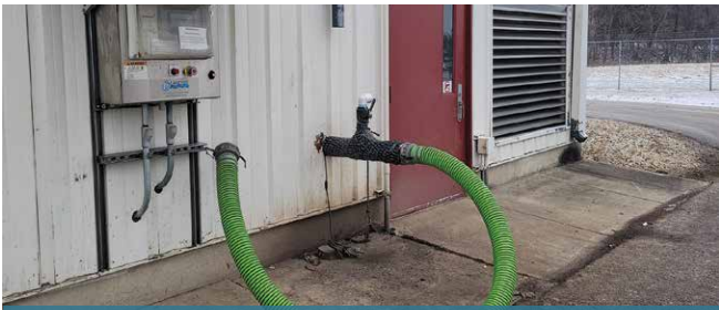
Septage haulers receive access by the plant's assigned PIN to activate the system.
