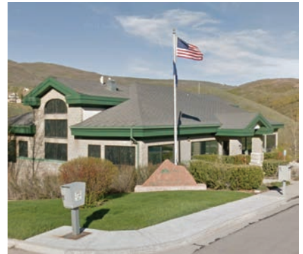
Snyderville Basin Water Reclamation District
