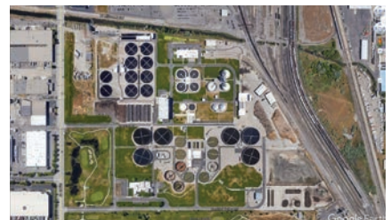
Central Valley Water Reclamation Facility
