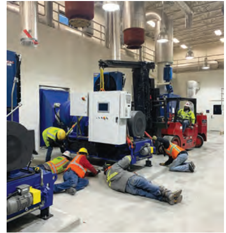
Archer Western installing new blowers at Timpanogos
