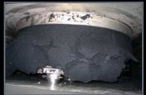
Dewatered Anaerobic Biosolids
